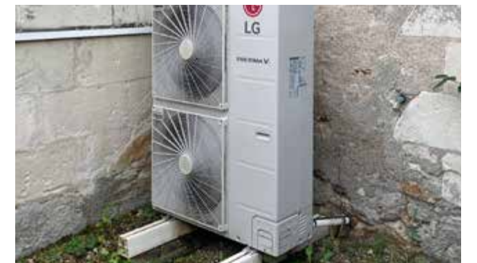
Example of a heat pump installation
